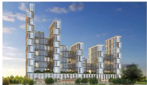
Sobha One achieved the prestigious BCA Green Mark Platinum Super Low Energy (SLE) Certification The First SLE Platinum outside Singapore
