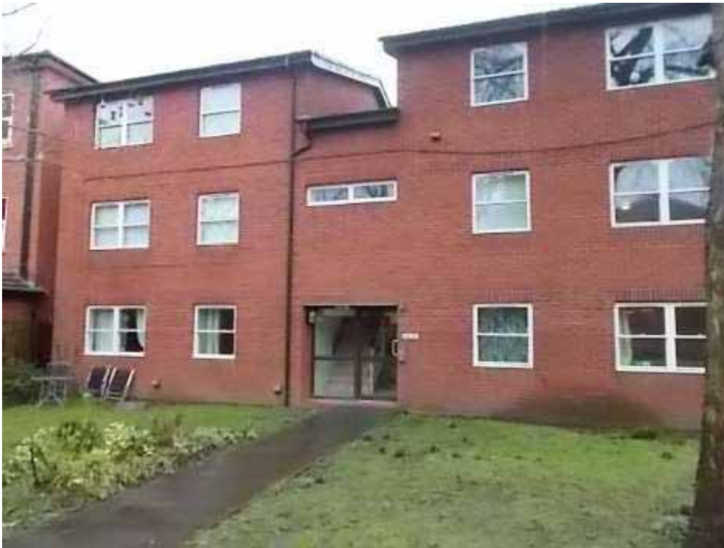
DE1 1HE, 23 Friargate Court, Friargate
