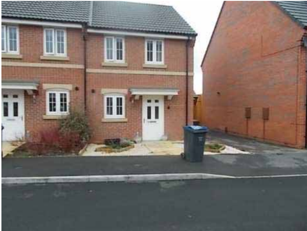
LE16 9FJ, 29 Bradford Street, Market Harborough
