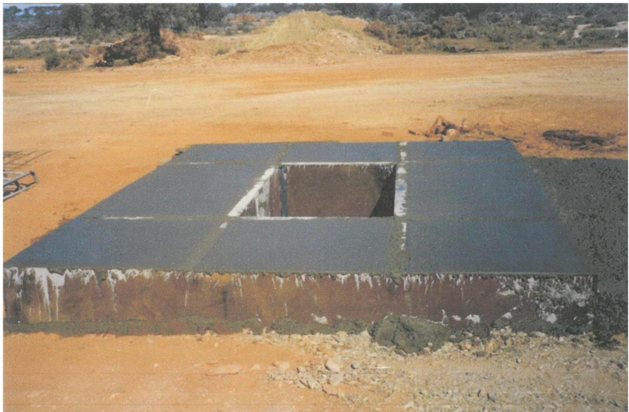
Figure 2. The new cement footing laid at the Eclipse shaft
