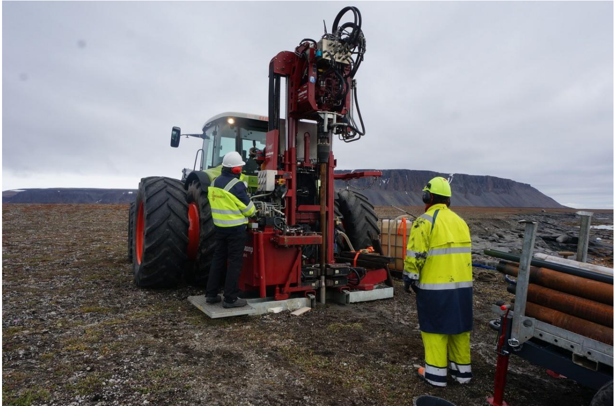
Figure 1: Sonic Drill Rig on Site at Thule Black Sands (July 2021)
