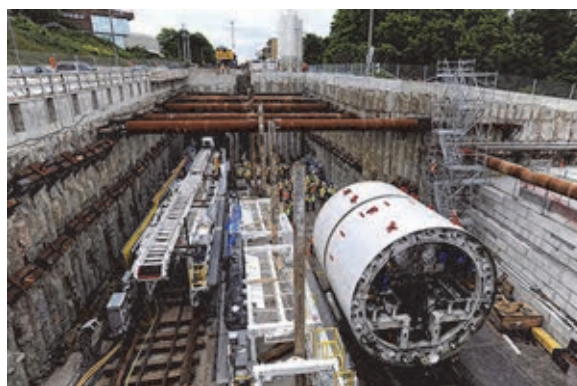
The tunnel-boring machine at the Eglinton Crosstown LRT construction site.
