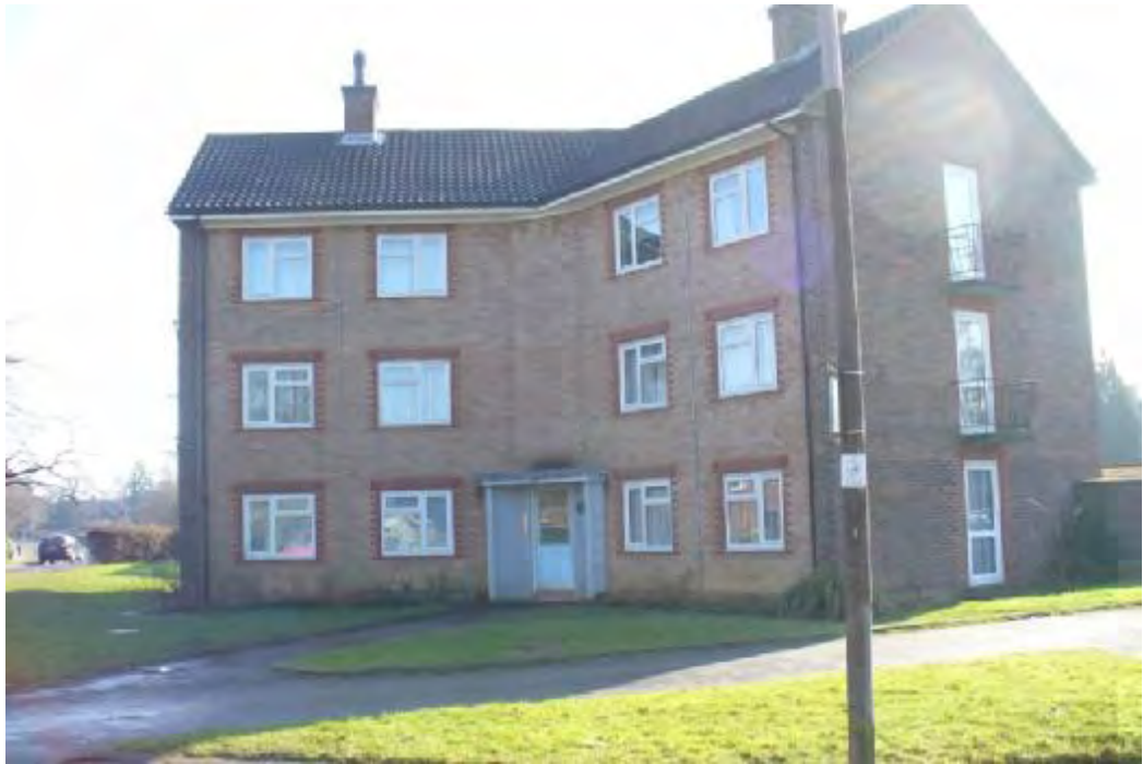
Flats 1-8 Aylwin Court, Granary Way, Horsham
