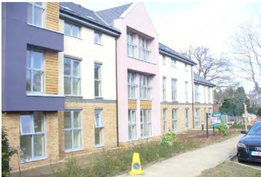
Leggyfield Court, Redford Avenue, Horsham
