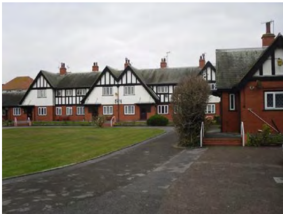
1-24 John Howard Cottages, Roedean Road, Brighton
