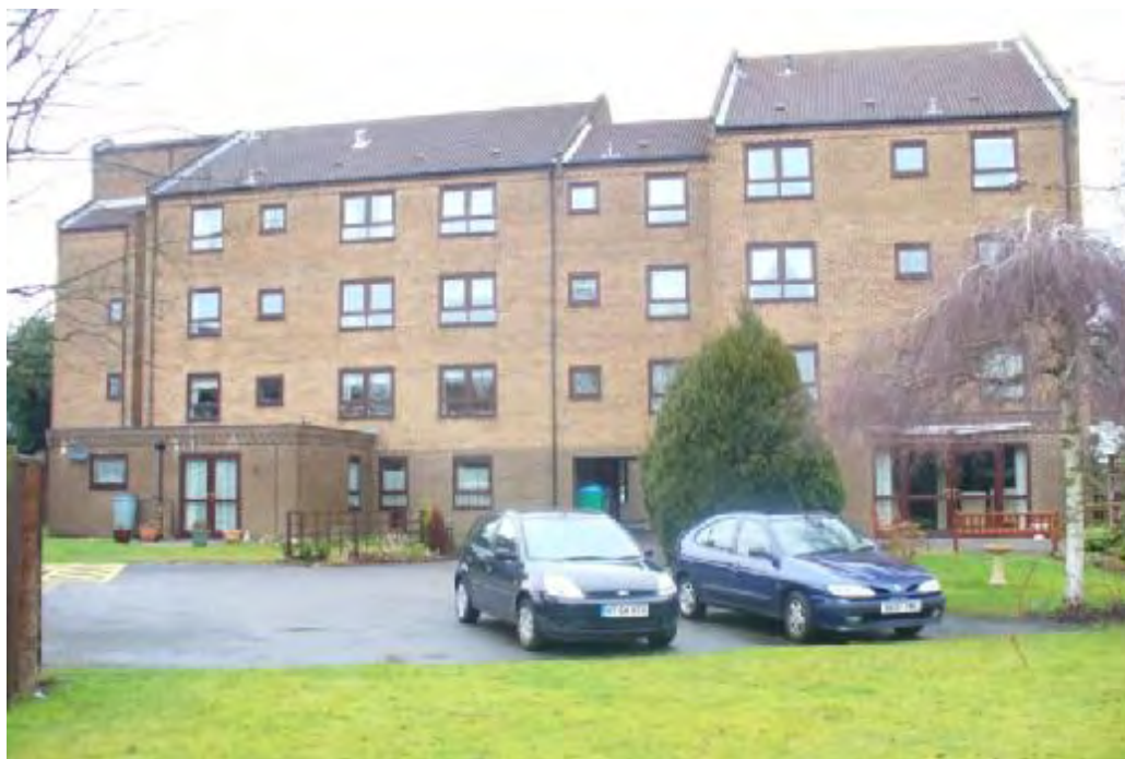
David Lockhart Court, Westwood Road, Southampton
