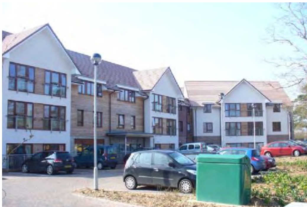
Abbotswood, Station Road, Rustington
