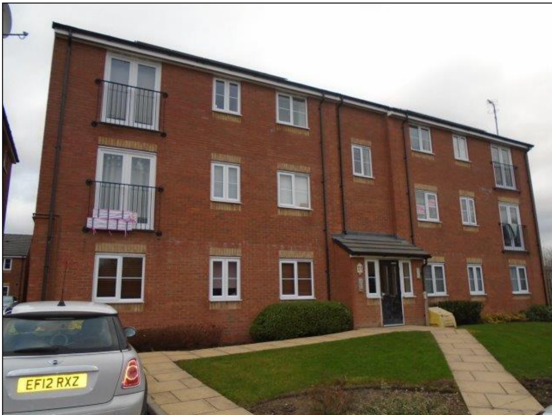
Swan Close, Bermuda Village, Nuneaton, Flats
