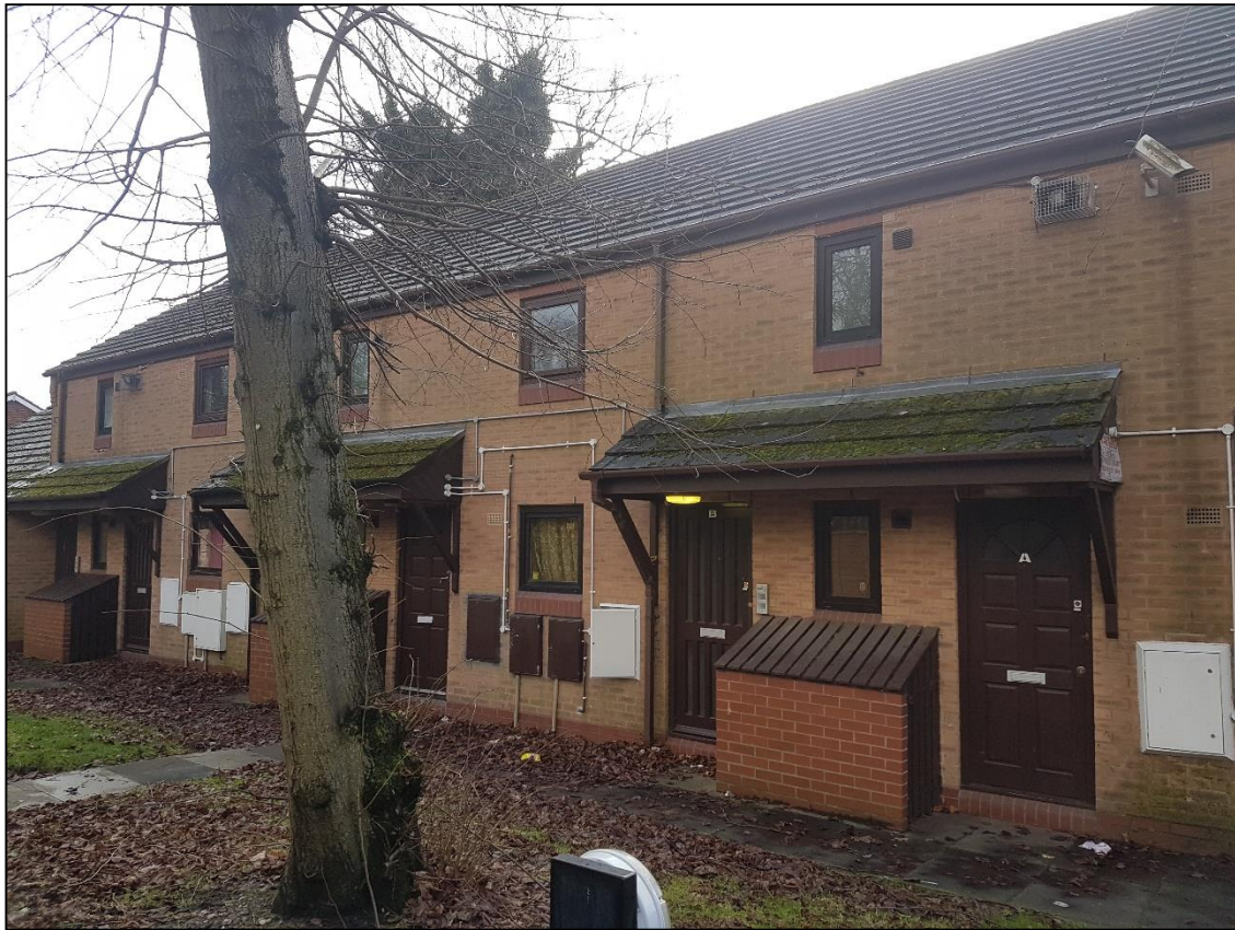
Rookwood Road, Acocks Green - No. 2, Flats A-G
