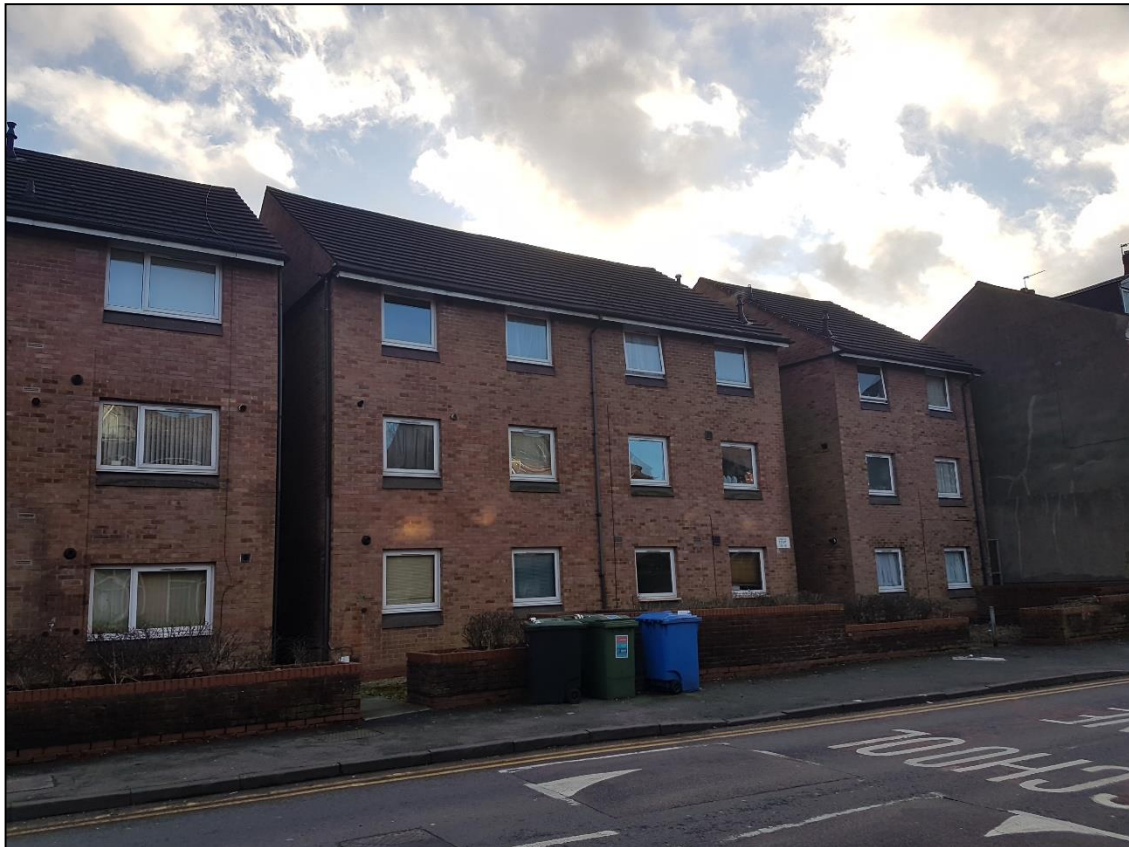
Gregg Court, Edgbaston Road, Balsall Heath - Flats 9-16
