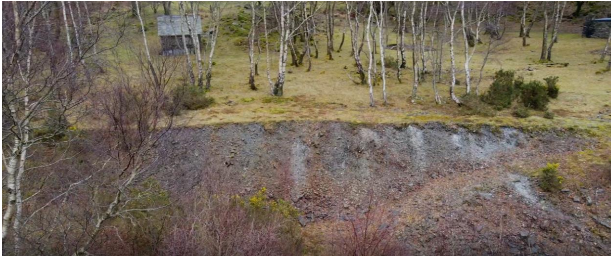
Figure 1: Aerial photograph taken from one side of the waste rock dump. Depth of waste rock dump shown is about 10 metres.
