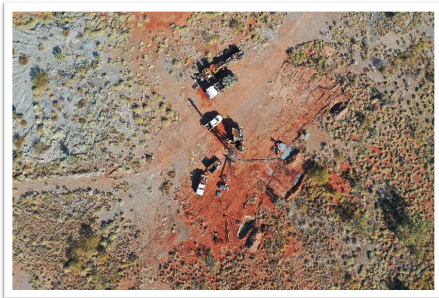
Figure 6: Birds eye view of drill rig set up, Elizabeth Hill, September 2021
