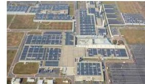
Solar panels at a new plant in China
