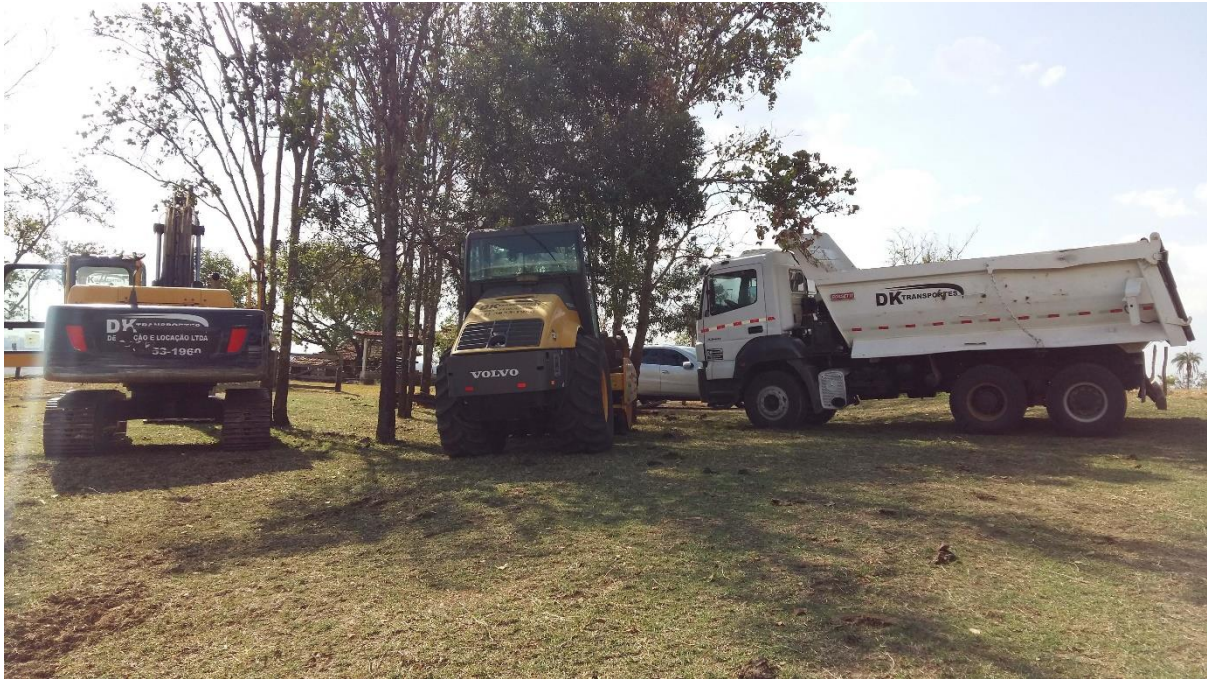
Figure 1: Initial Plant Arriving at Site
