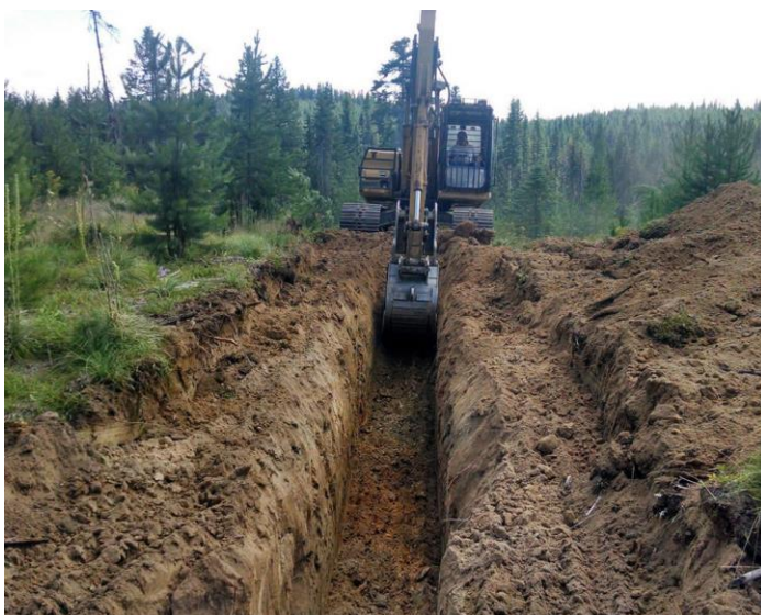
Figure 3 (left): Trenching to expose bedrock (not Clogau)
