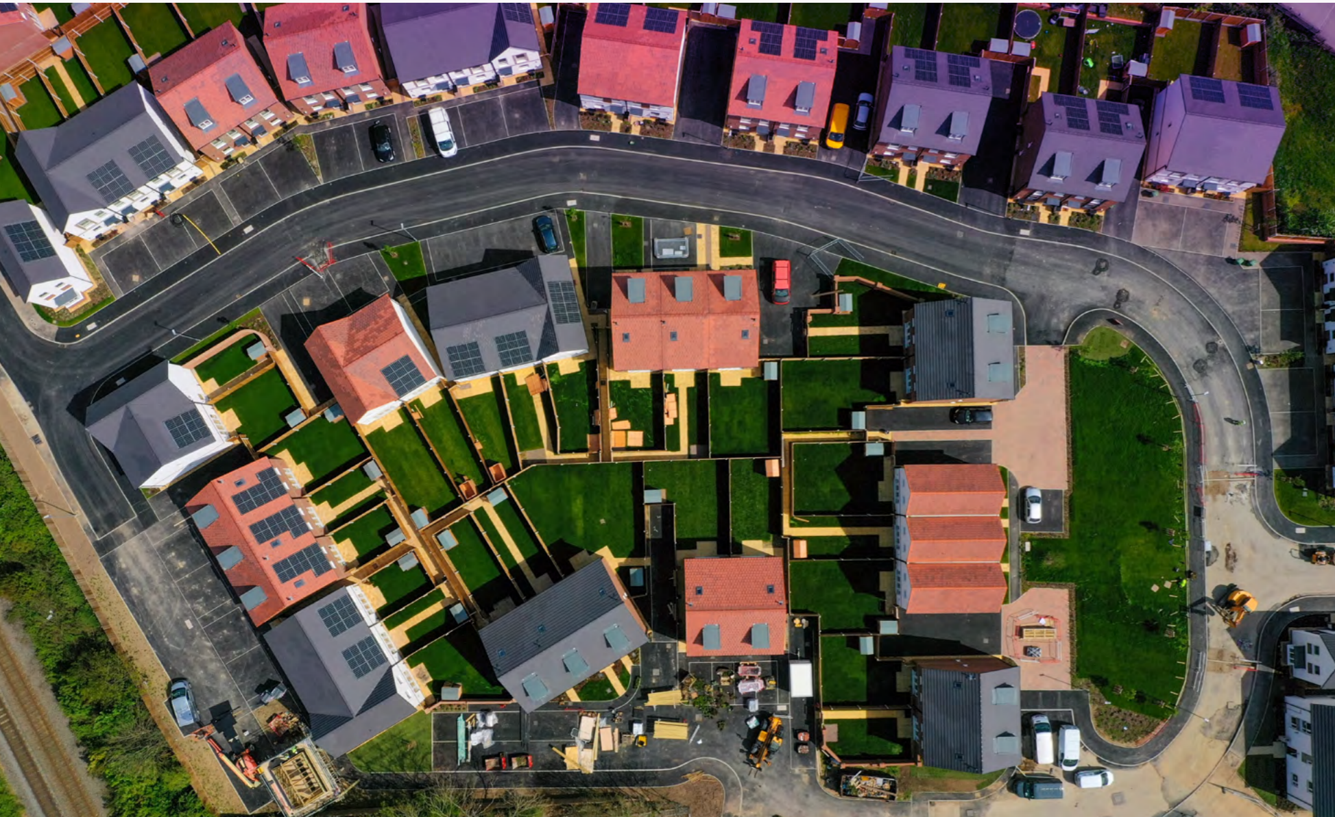
↑ Pictured: Green Vale development, Worcestershire
