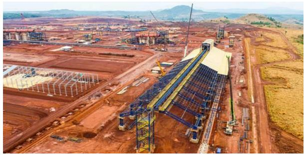
All the structural steelwork is in place on the ore homogenisation building, with the cladding of the roof underway.
