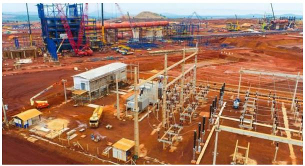
The Araguaia sub-station with both of the main 230kV/34.5kV transformers installed.
