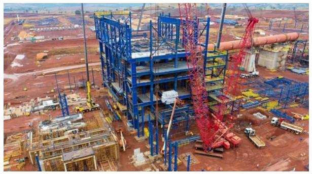
The Electric Arc Furnace building in the centre with the electrical transformer being positioned on the second level, to the left of the image is the refinery building.
