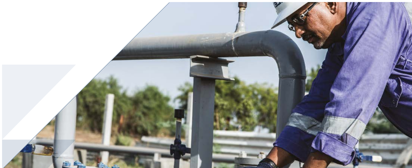
Figure 4: Oilex Staff at Cambay Production Facility
