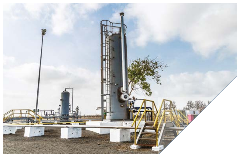
Figure 5: Bhandut Production Facility
