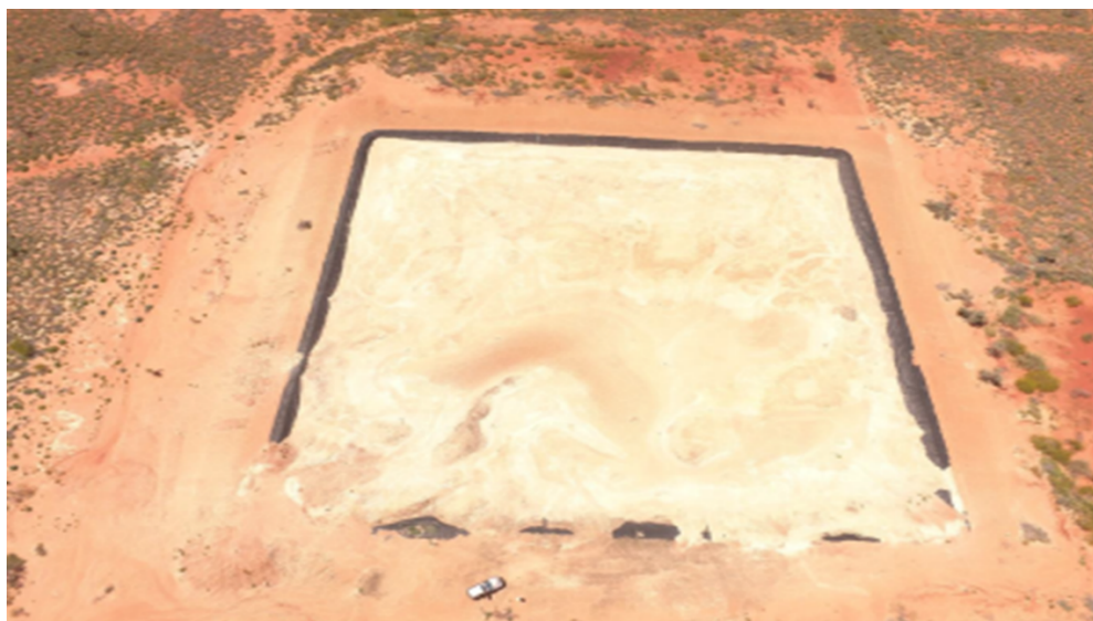
Figure 2: Tailings Dam, Elizabeth Hill Silver Project, June 2021
