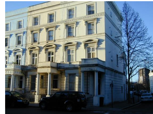
Ladbroke grove 129 W11
