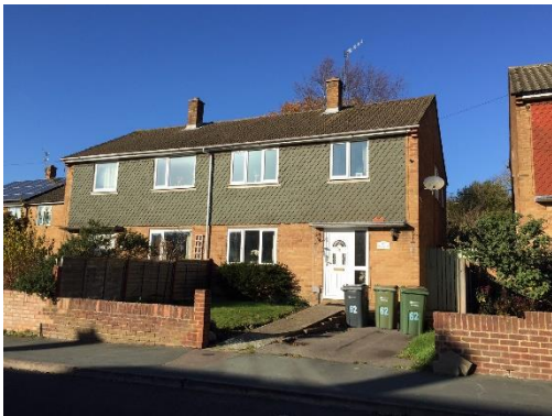
Fairview Road, Ash, 62
