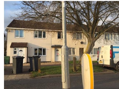
Oakridge Road, Basingstoke, 19
