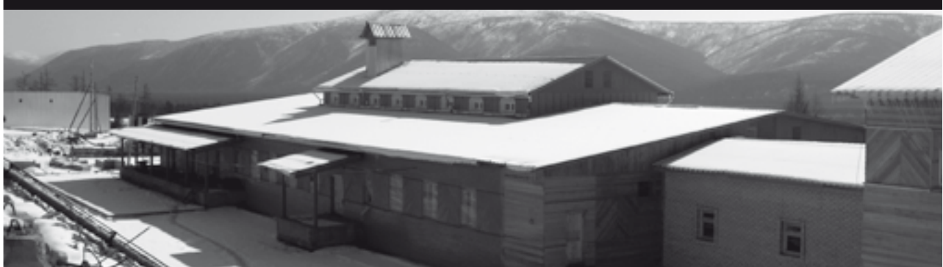
Accommodation block at Kuranakh
