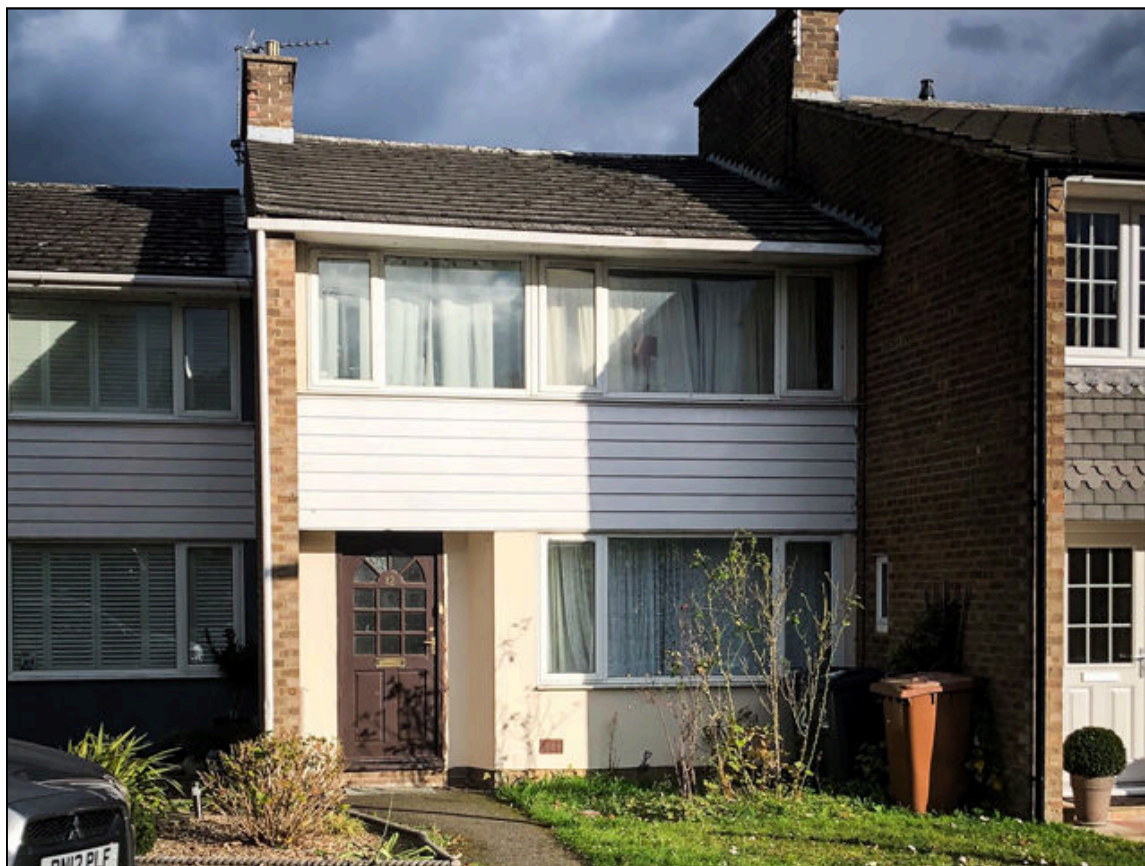
SG9 9NN, 12 Bridge End
