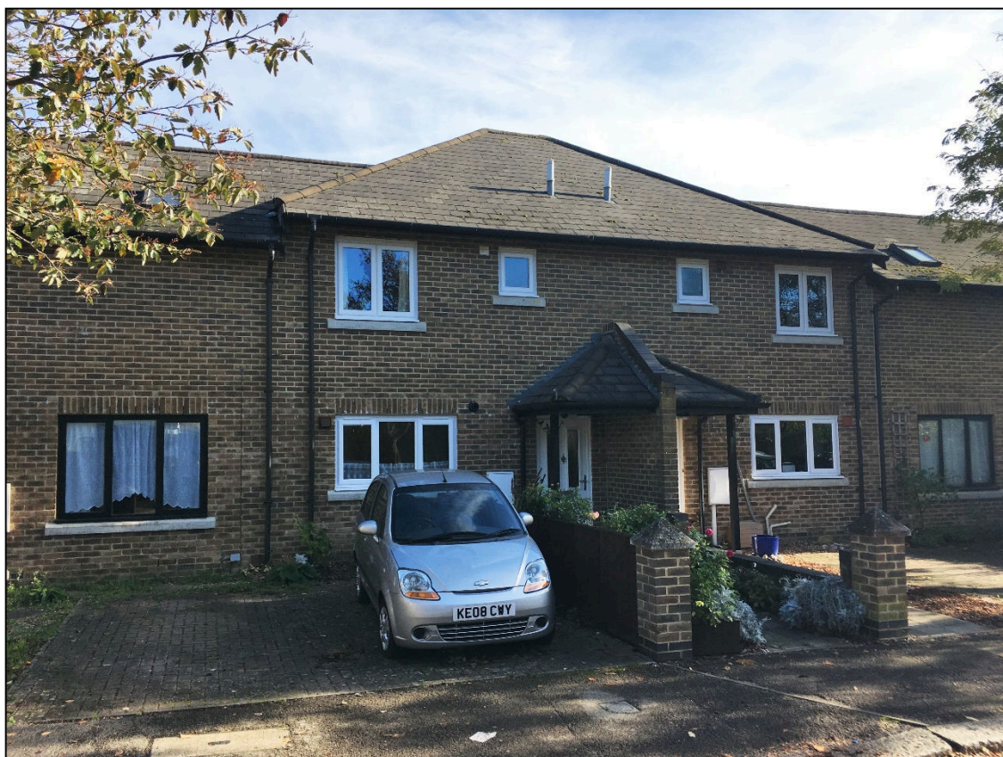
TW11 0QE, 86 Kings Road
