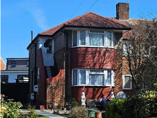
HA0 2HF, 25 Fernwood Avenue Sudbury
