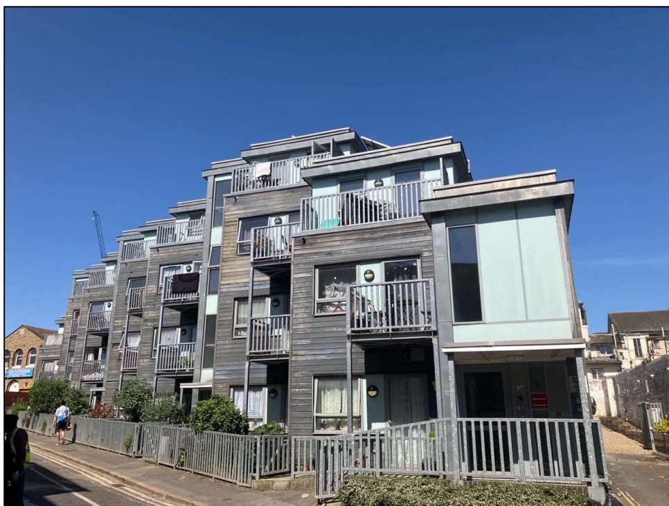
CR0 3LE , FLAT 2 Baker House Handcroft Road Croydon Surrey
