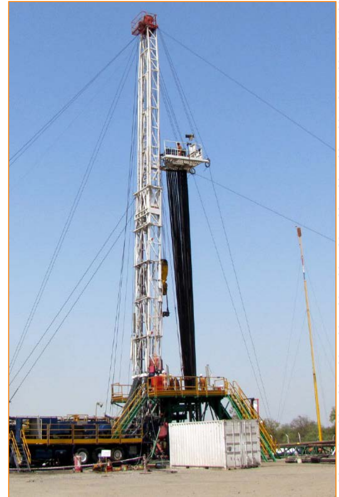
Workover rig operations
