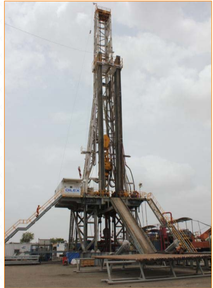
Rig at Cambay-76-H
