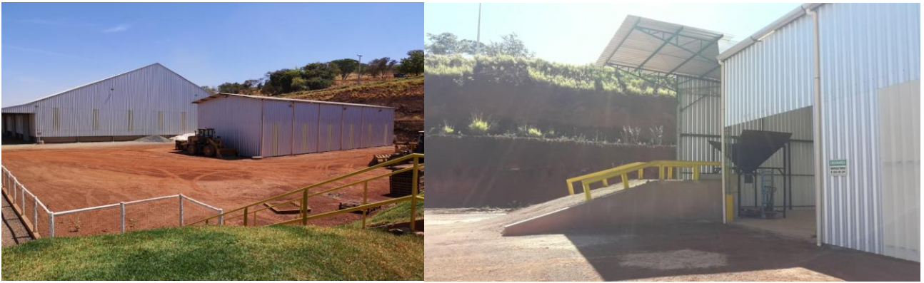
Figure 1: New “Big Bag” storage facility and loader
