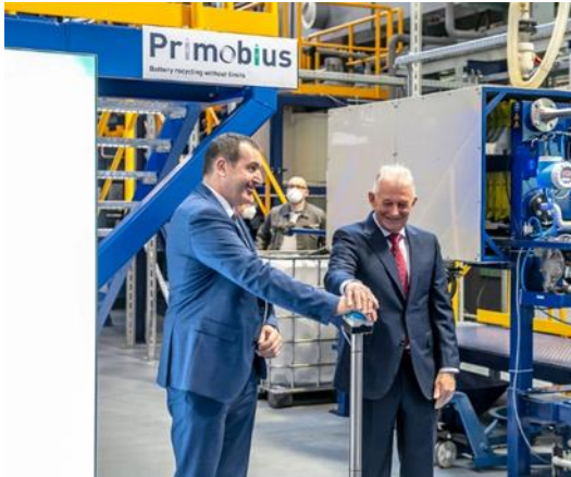
Figure 3 – Primobius Managing Directors Horst Krenn and Michael Tamlin (l-r) officially open the 10tpd Shredding Plant
