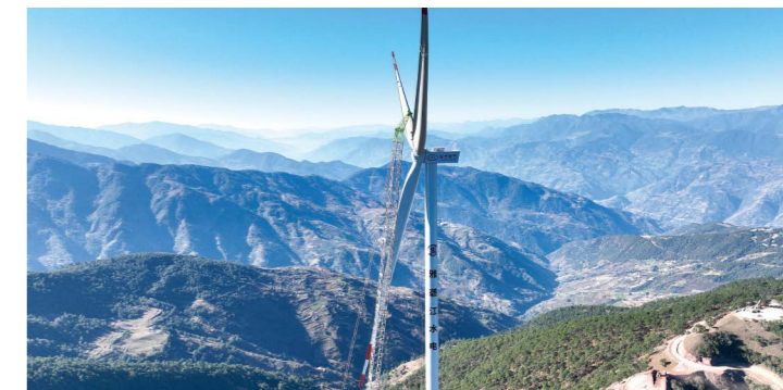
▲ Hoisting of the first wind turbine on Laba Mountain
