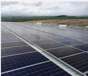
iDube Cold Storage
