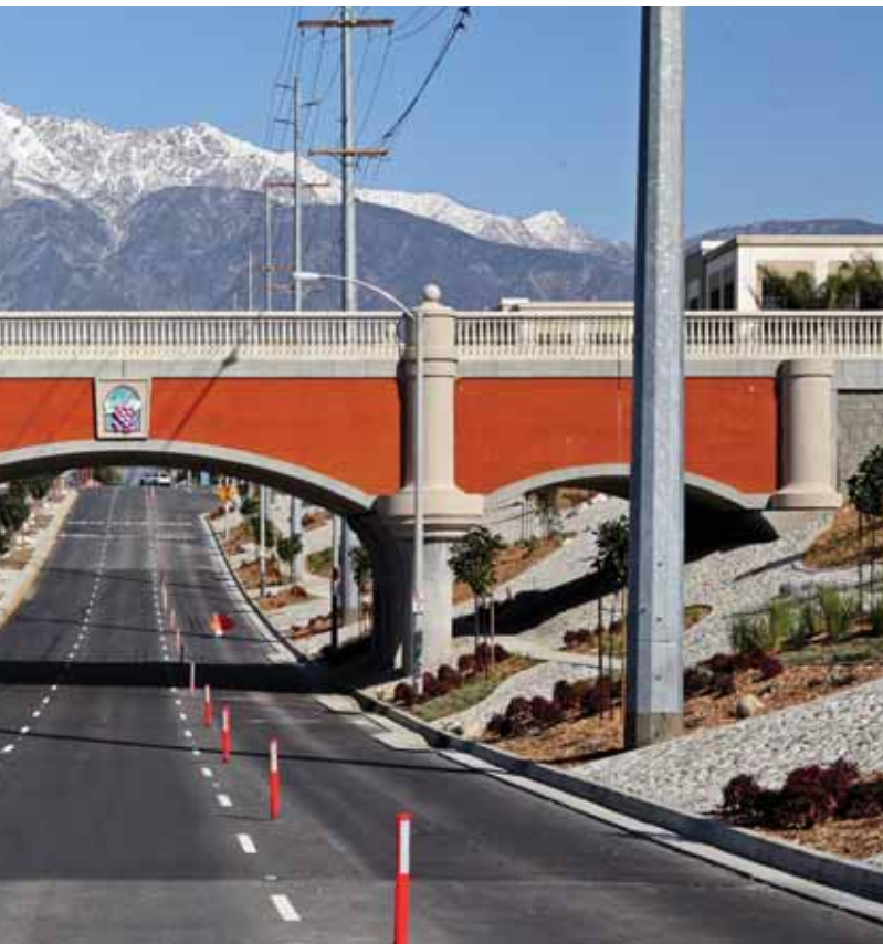
Oldcastle Precast developed prestressed concrete post-tension box girders for the City of Rancho Cucamonga outside of Los Angeles, California. The bridge includes a 33-foot and a 52-foot girder, together carrying two railroad tracks over Haven Avenue.
