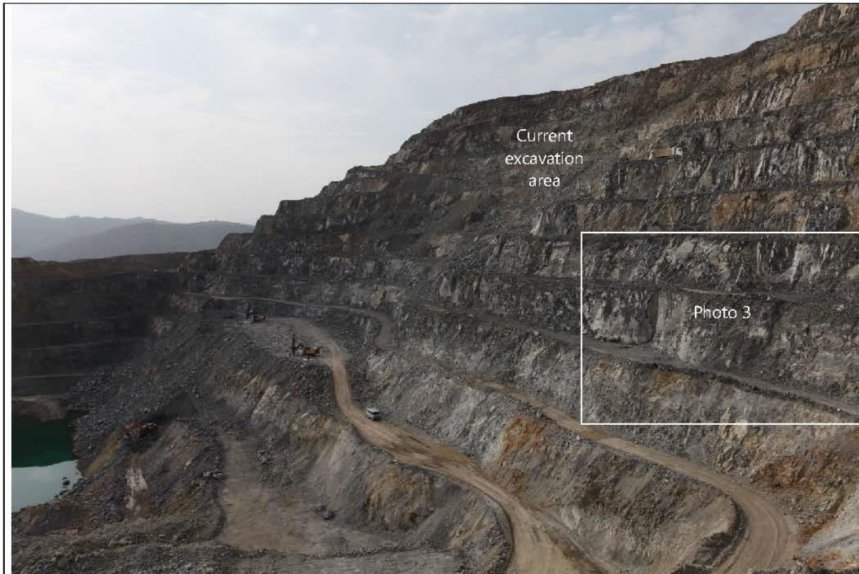
Photo 2 Pit slope with current excavation zone Location of Photo 3 is indicated
