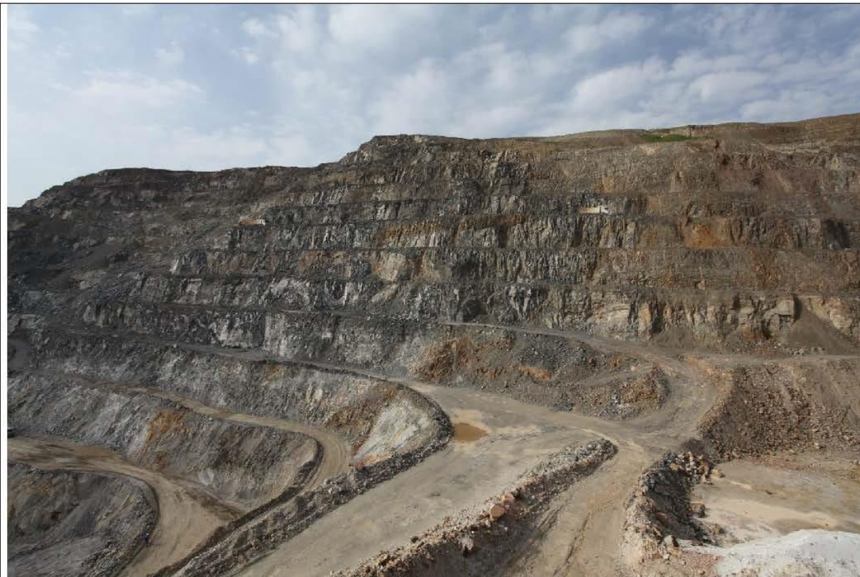
Photo 1 General view of pit slope
