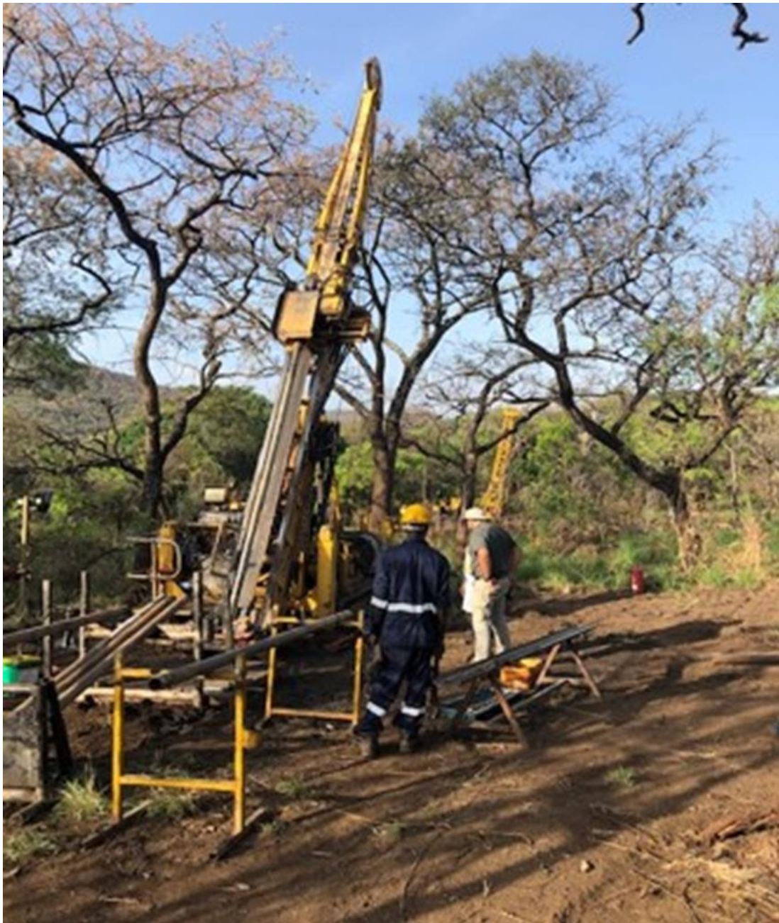
Figure 3: Drill rigs on site March 2020
