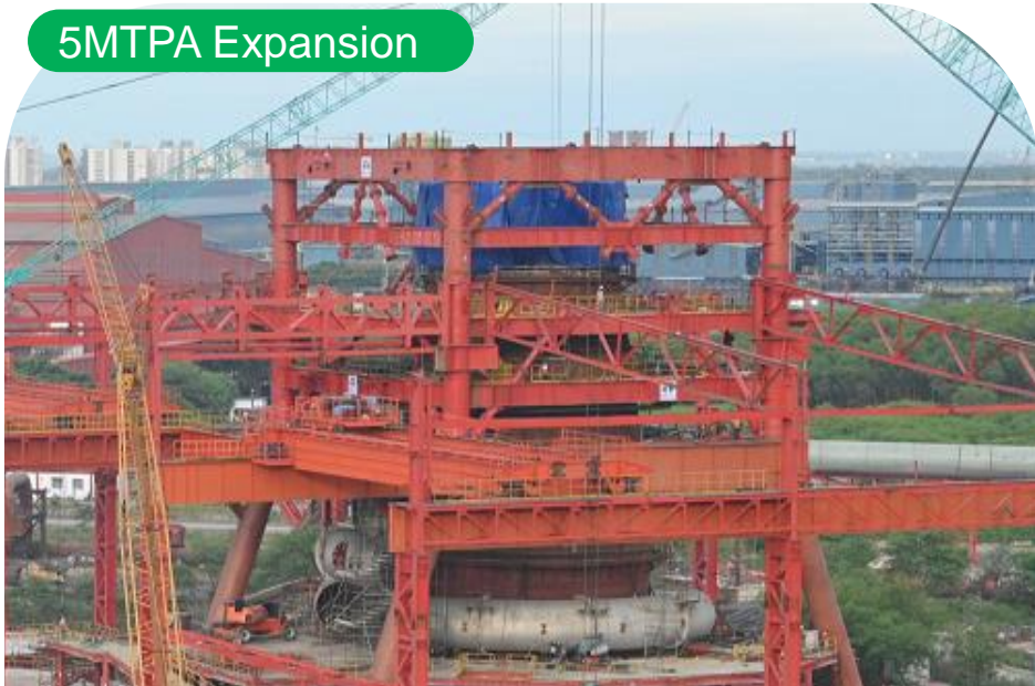
Outer shell of Blast Furnace has been erected
