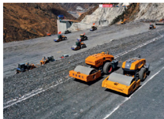
▲ Intelligent Unmanned Roller for Dam in Operation
