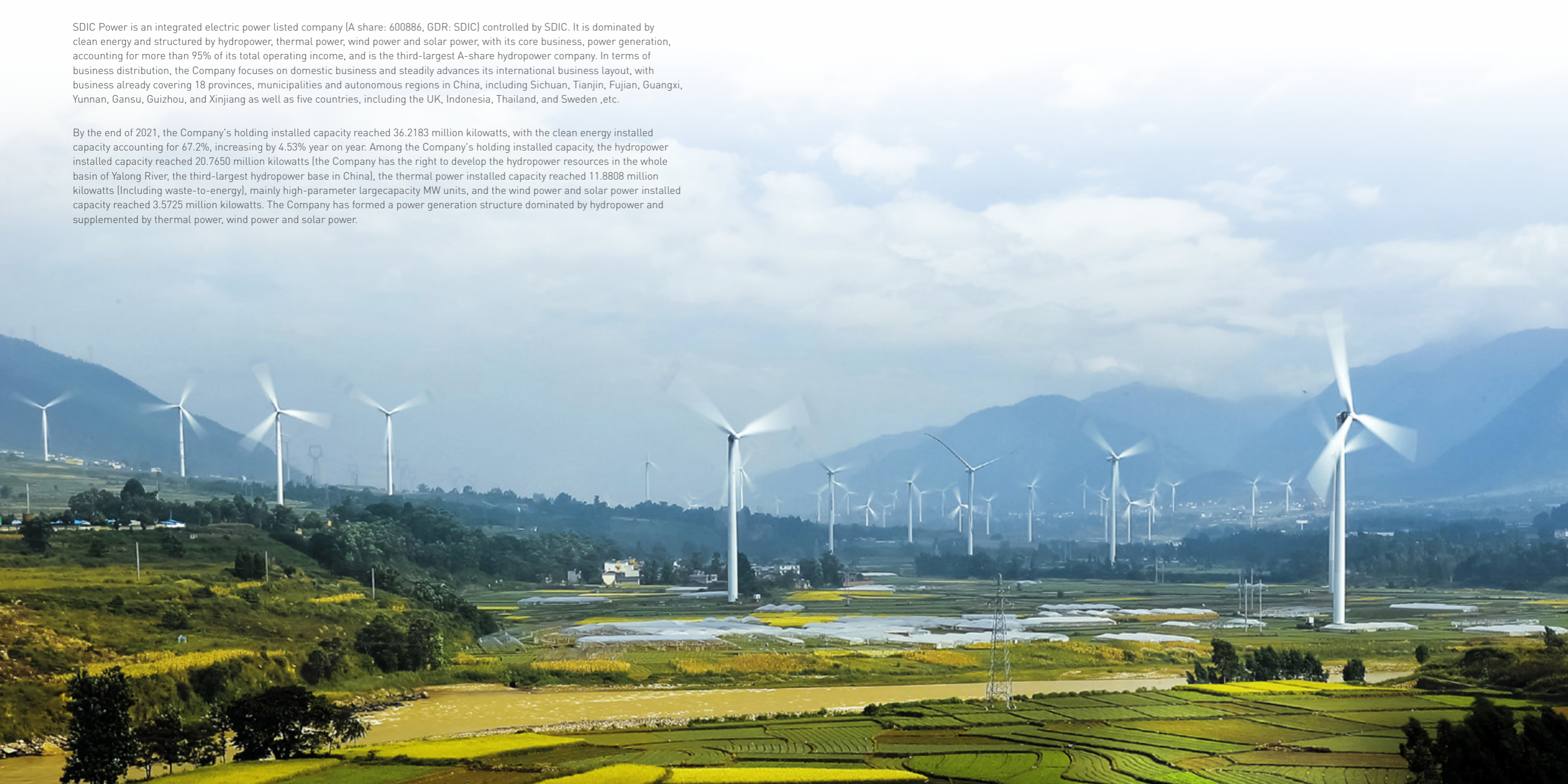
▲ Dechang wind power of Yangfanggou Hydropower Station, Sichuan
