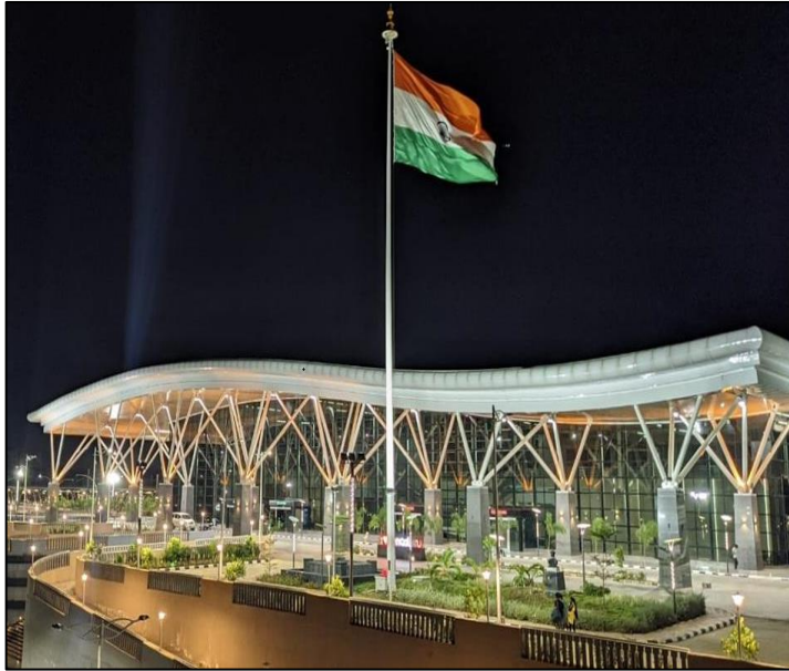
Tata Structura used at Sir Visvesvaraya Railway Terminal, Karnataka
