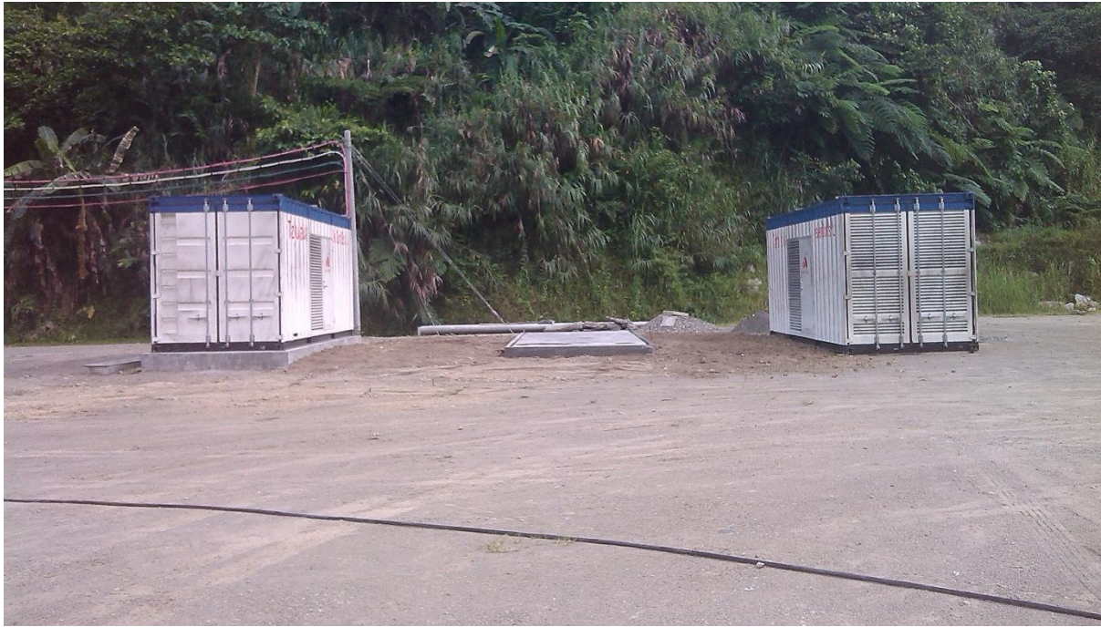
Image 7. Construction generating capacity – Two 1,000 kVA units
