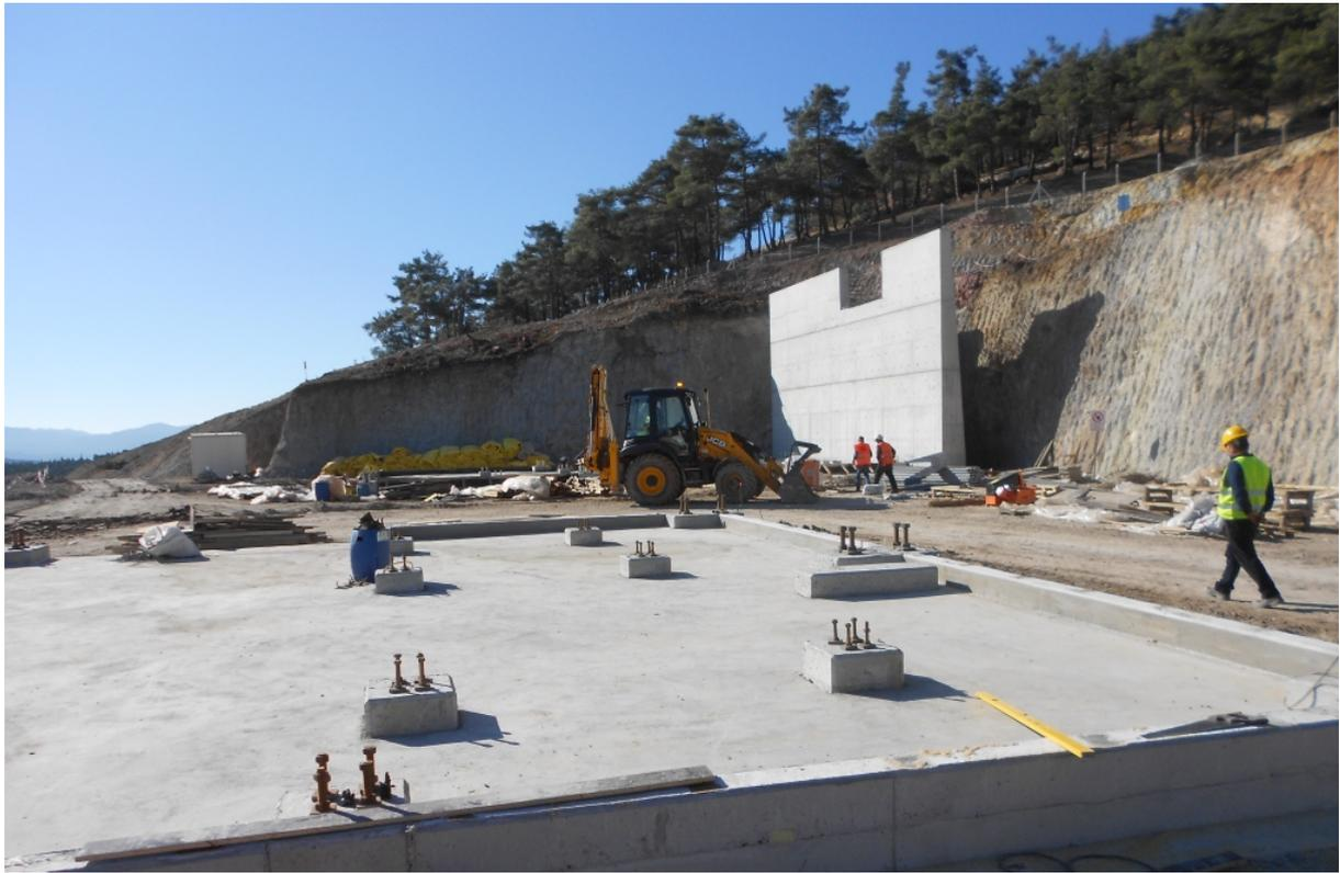
**Figure 2:** Crushing unit foundations ready for the mounting of structural steel and crushers.
