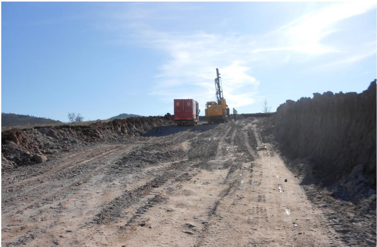
**Figure 3:** Open-pit entry ramp at Arzu South being prepared for its first blast.
