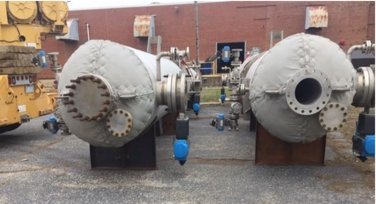
Figure 3: Test Reactors being staged for installation
