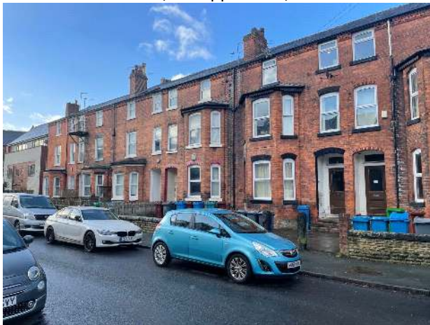
M21 0AT Flat 1, 11 Keppel Road, Manchester
