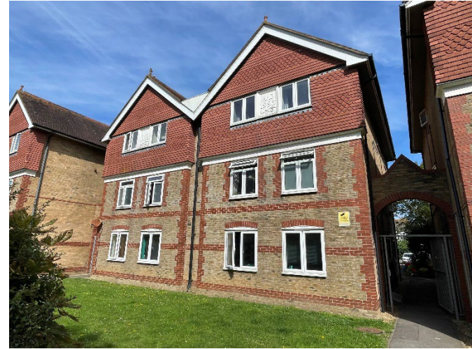
East Hill Court, Worthing
