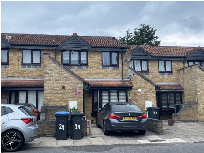
Dickenson Close, Edmonton
