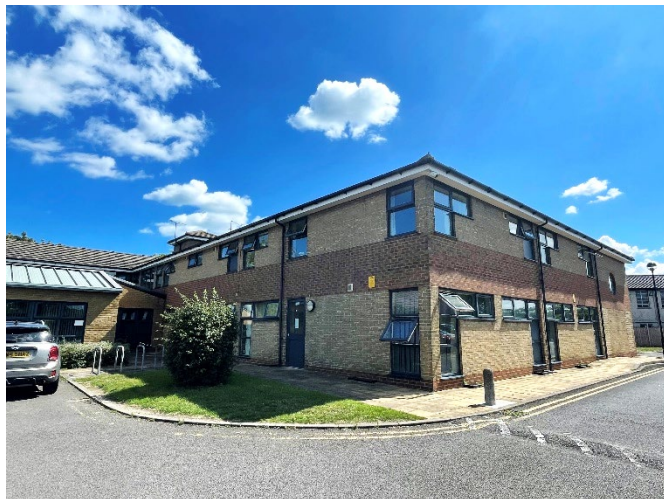
Bridge House, Sheerness
