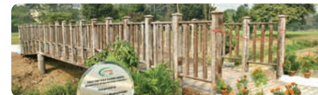
Bridge at Golmuri Golf Club in Jamshepdur made of Fibre Reinforced Polymer (FRP) Composites
