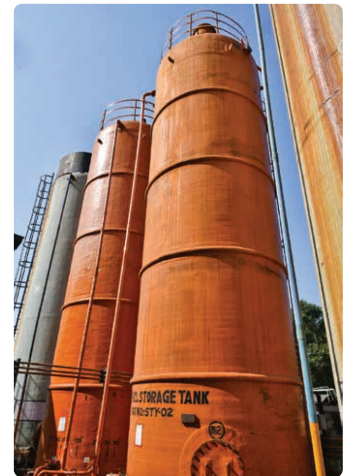
Storage Tanks made of Fibre Reinforced Polymer (FRP) Composites
