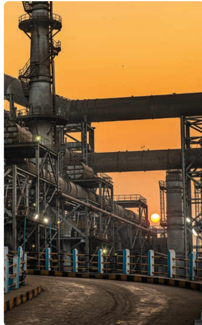
Blast Furnace, Tata Steel Meramandali Works
