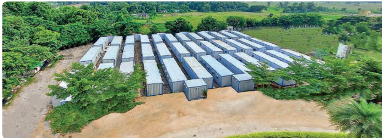
Tata Steel Medica Hospital, Odisha constructed using Nest-In MobiNest solution. The 156-bed 25,578 sq. ft. hospital was constructed as part of Tata Steel's COVID-19 response
