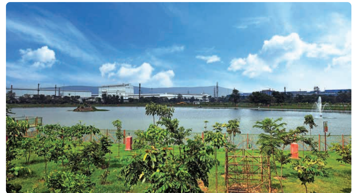
Rejuvenated CRM Bara Pond at Jamshedpur, Jharkhand
