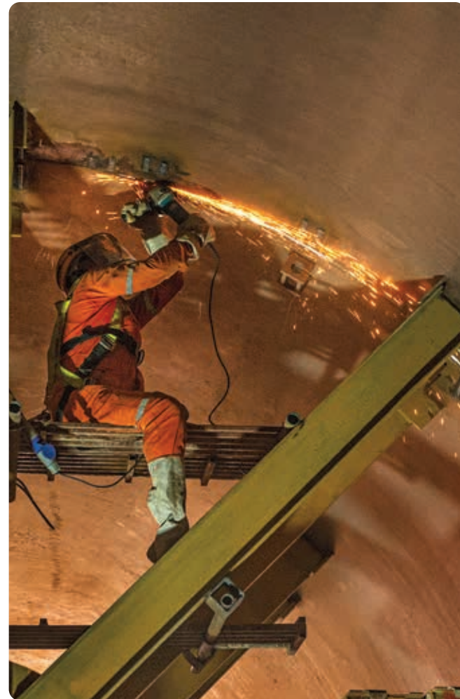
Blast Furnace, Tata Steel Kalinganagar Works
