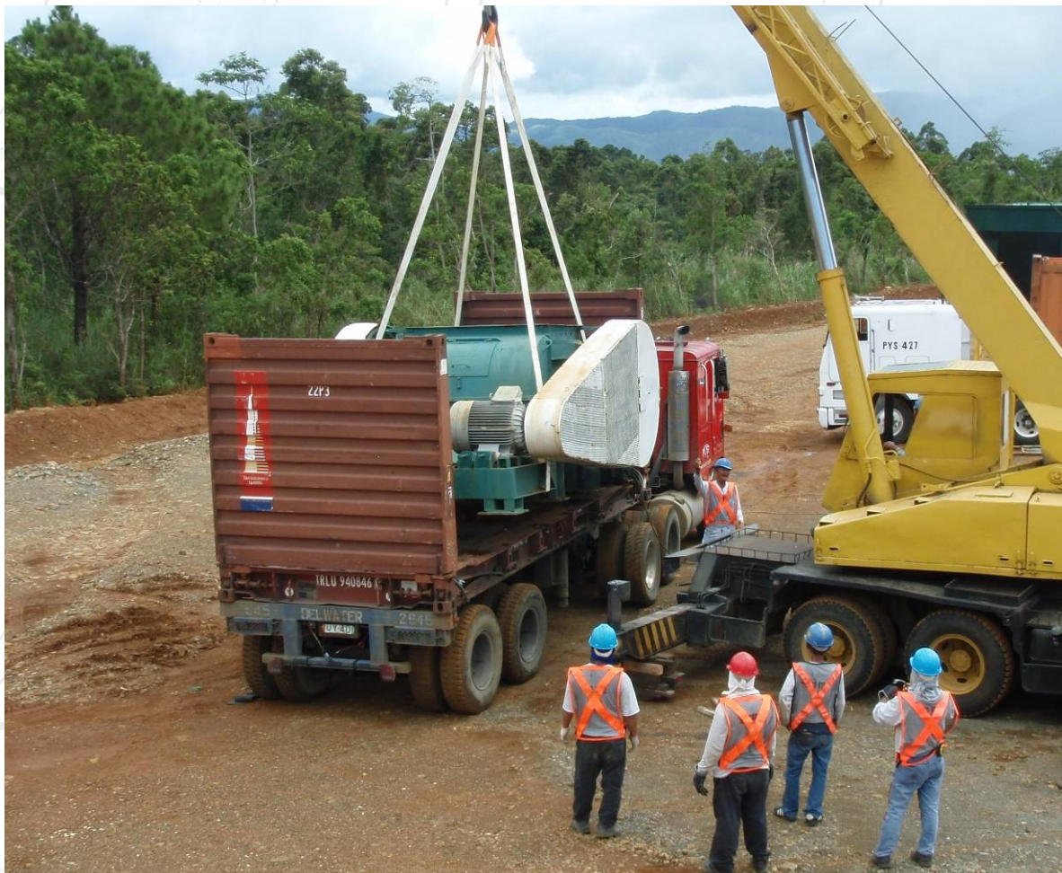
..... Fig. 1: Crusher being unloaded at trial heap leach site. ....
