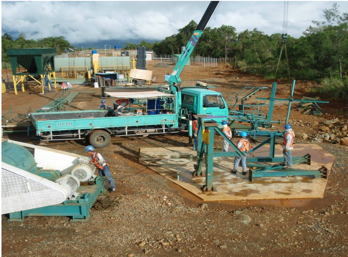
Fig. 2: Crusher under construction at trial heap leach site.
