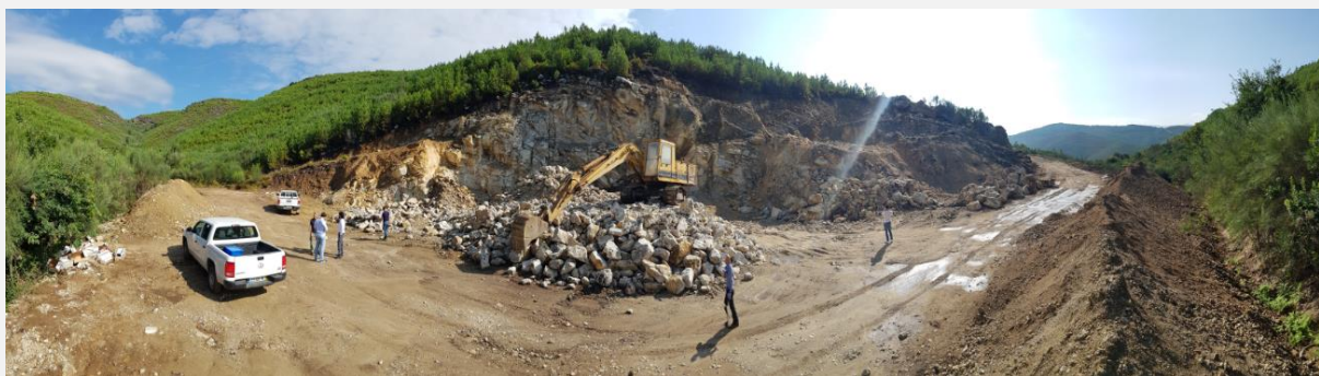
Figure 5. Photograph of the Quarry
