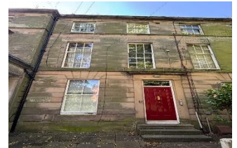
CH43 4UP, 27 DEVONSHIRE ROAD_FLAT 2, PRENTON, WIRRAL
