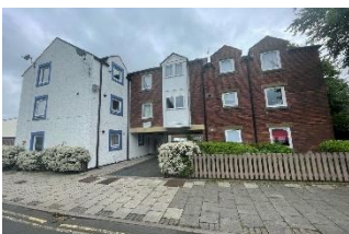
CA2 5XF, 81 MILBOURNE STREET, CARLISLE
