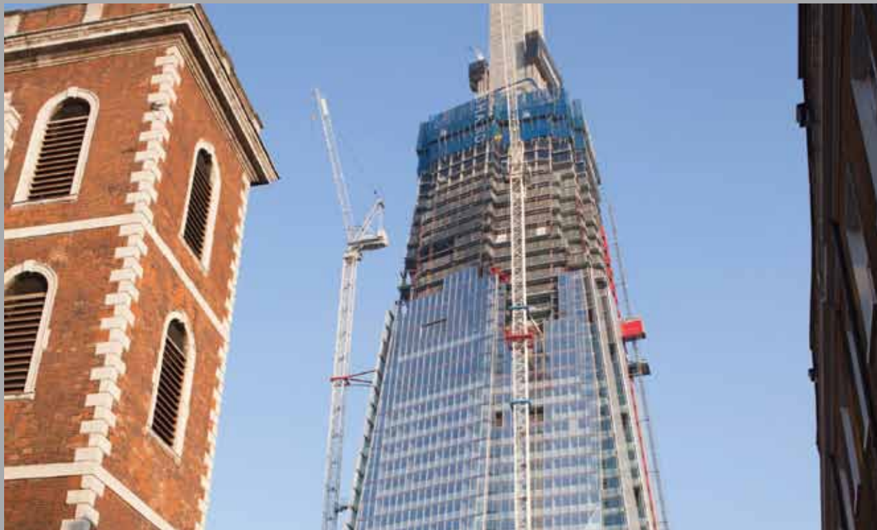
PROJECT → The Shard LOCATION → London Bridge
