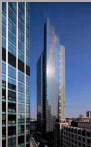
PROJECT → Heron Tower LOCATION → London
