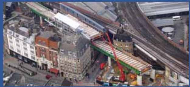
PROJECT → Thameslink Borough Viaduct Bridges LOCATION → London
