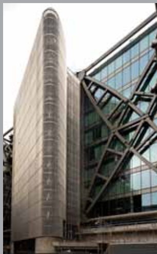
PROJECT → Cannon Place LOCATION → London
