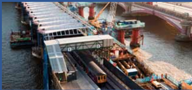
PROJECT → Blackfriars Bridge Deck Replacement LOCATION → London
