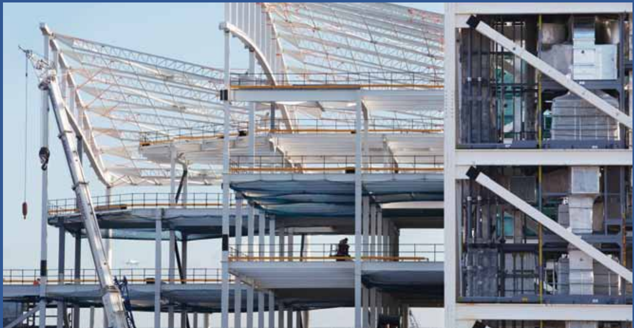
PROJECT → Heathrow Terminal 2A
