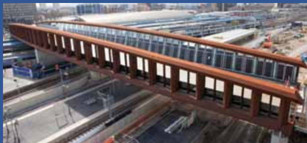
PROJECT → Link Bridge LOCATION → Stratford City, London
