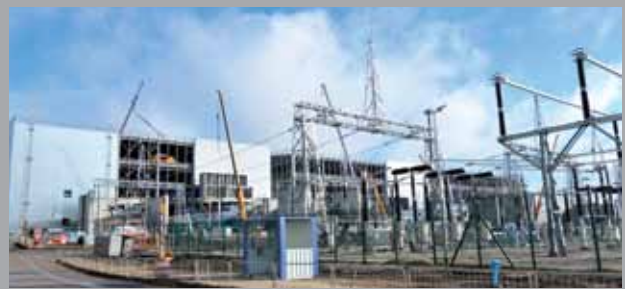
PROJECT → West Burton Power Station LOCATION → Retford
