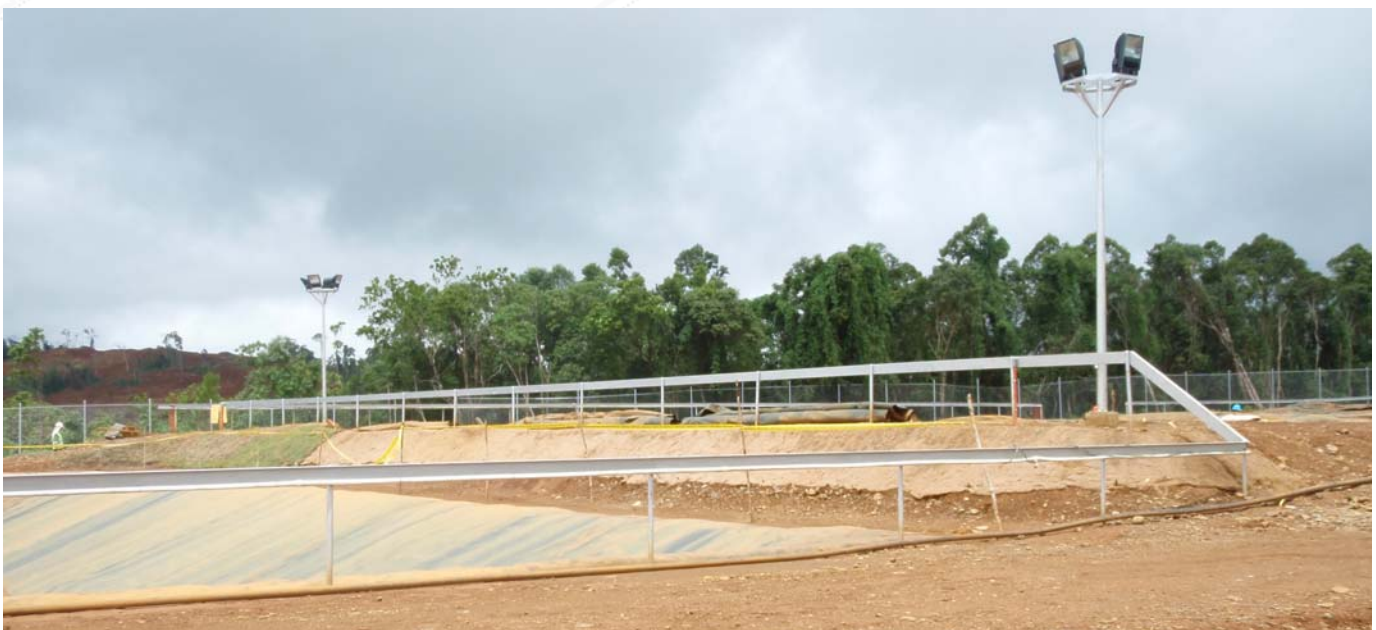
Fig 1 : HLT Pregnant Leach Solution pond. This has a floating raincoat that creates a closed system with the Heap Leach Pad on the upper level to the right of picture. The Heap will also have a raincoat once the agglomerated ore is placed later this quarter.
