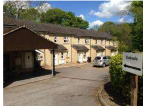
Oakvale House VG 29
