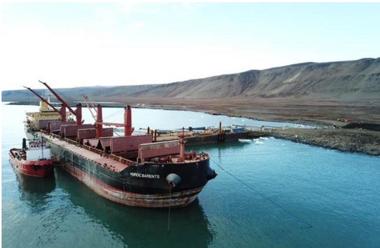
Figure 5 – Loading of bulk carrier. Direct shore loading should allow for significant capex reductions.
