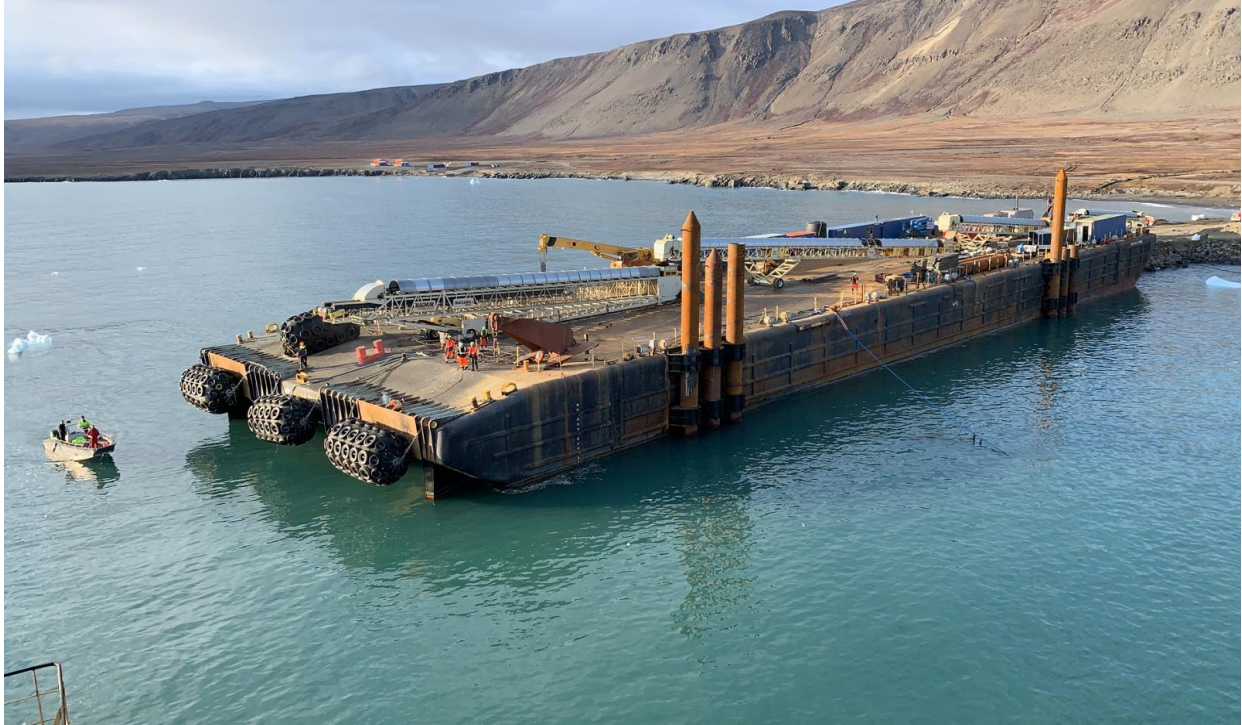
Figure 3 – Barge loading platform.
