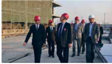
Rudy Markham and Oliver Stocken visit the construction site of our new building in Tianjin
