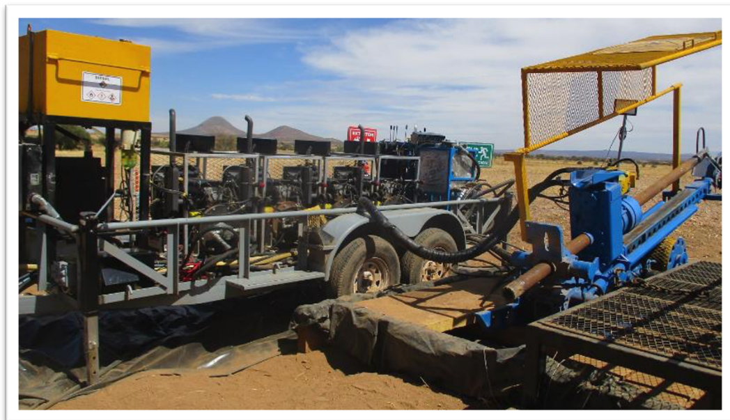
Figure 3: Ecodrill Hydracore Diamond Drill rig, Donovan 2, February 2021
