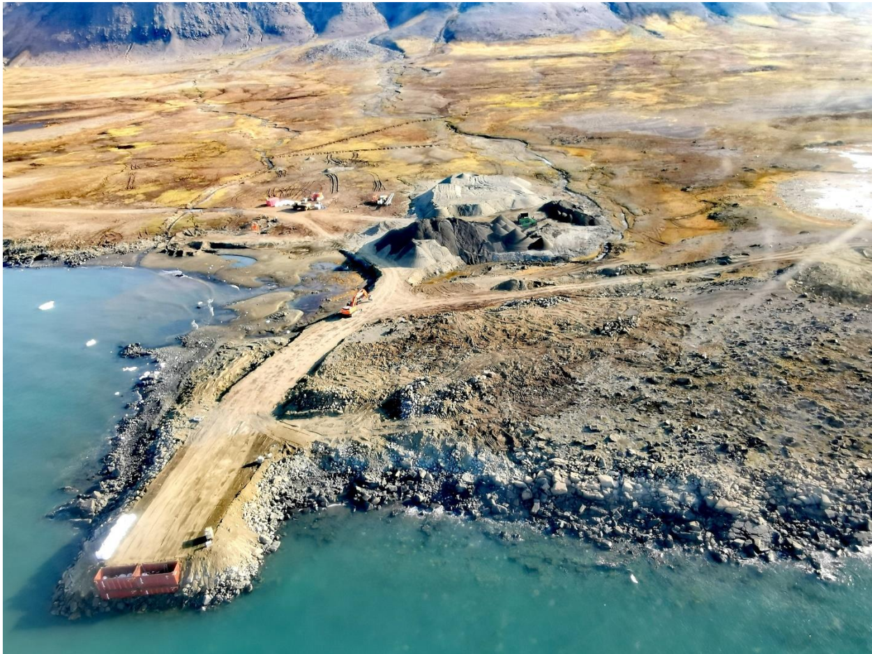
Figure 3 - Causeway constructed at Moriusaq in preparation for the ship loading operation
