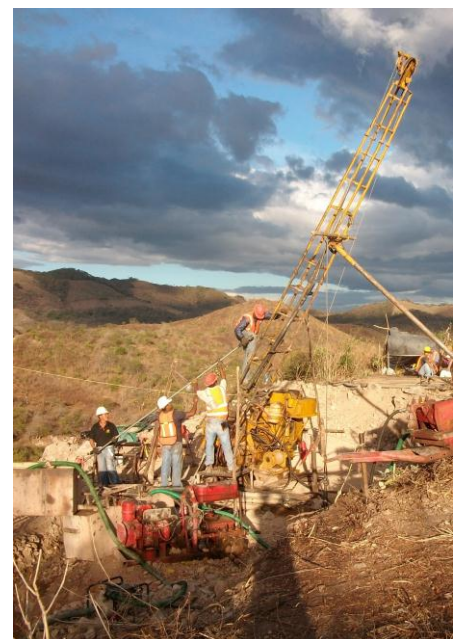
Diamond core drilling on the La India Project.
