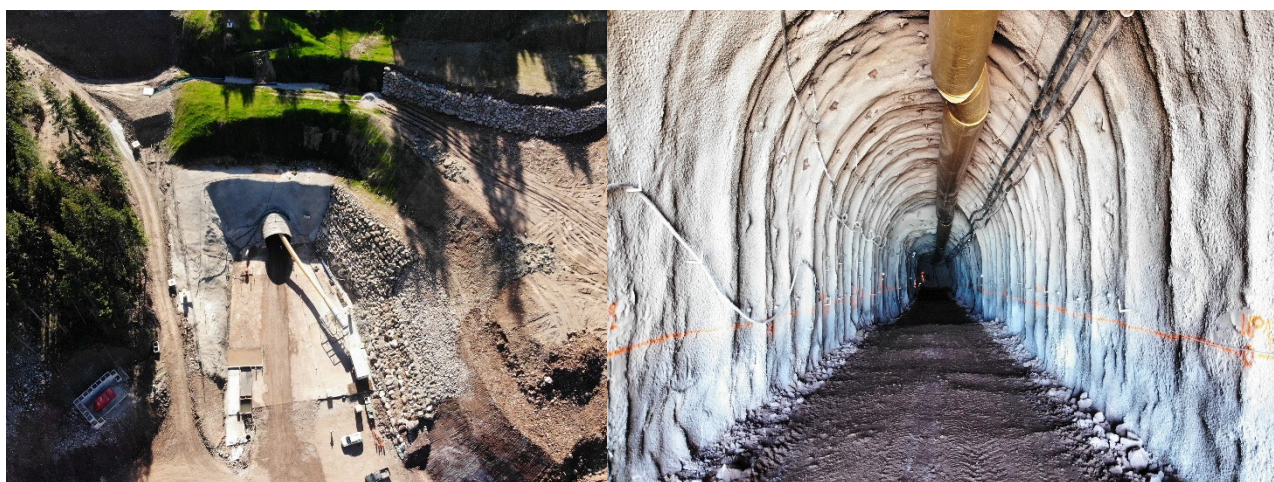
Figure 2: Upper Decline Portal and Underground Development
